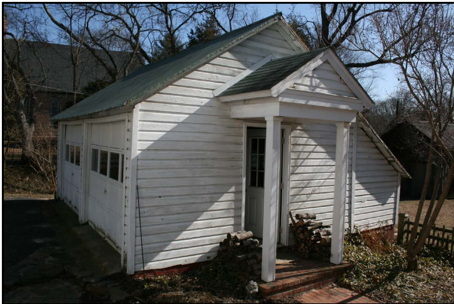
Photo: Garage, Upper Marlboro, view looking east. (February 2009)
