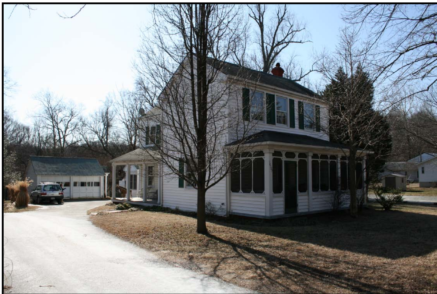
Photo: Bunnell-Anderson House, Upper Marlboro, side (north elevation), view looking southwest. (February 2009)
