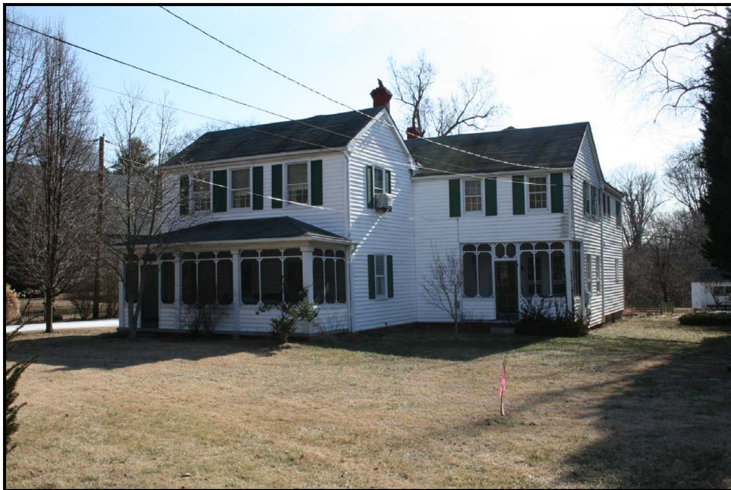
Photo: Bunnell-Anderson House, Upper Marlboro, side (north) elevation, view looking southeast. (February 2009)
